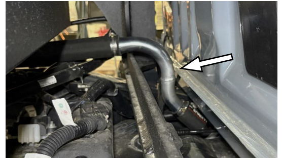
Photo 10: Install Steel Filler Neck
