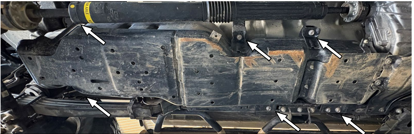
Photo 2: Remove OE Fuel Tank
