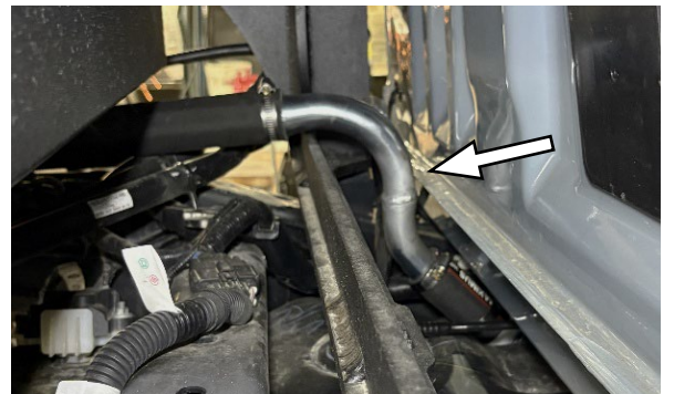
Photo 6: Install Steel Filler Neck
